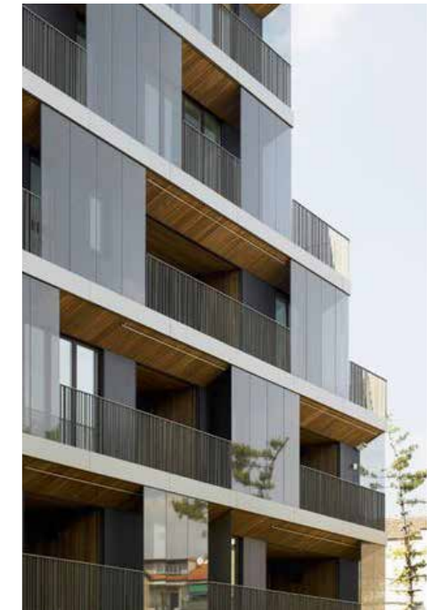
Metal balustrades to balconies
